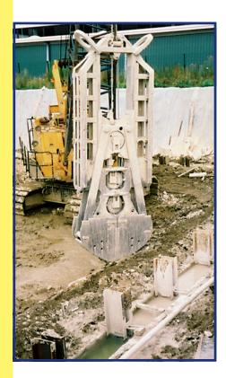
The cutting edges of the grab jaws are made of Hardox steel 450 and were especially hardened. Easy mounting of the grab jaws for excavation widths 600/800 mm. All the grab teeth as well as all the wire rope pulleys are quickly exchangeable due to their construction as ready to use components.
