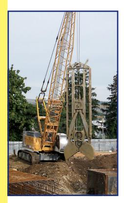
The cutting edges of the grab jaws are made of Hardox steel 450 and were especially hardened. Easy mounting of the grab jaws for excavation widths 500/600/800mm. All the grab teeth as well as all the wire rope pulleys are quickly exchangeable due to their construction as ready to use components.
