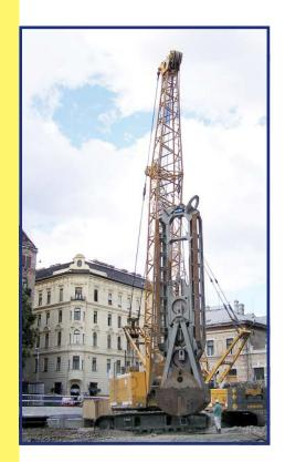
The cutting edges of the grab jaws are made of Hardox steel 450 and were especially hardened. Easy mounting of the grab jaws for excavation widths 1200/1300/1500 mm. All the grab teeth as well as all the wire rope pulleys are quickly exchangeable due to their construction as ready to use components.
